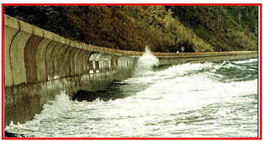
Protection walls are typically for coastal protection where wave loading, scouring and overtopping are key factors.
