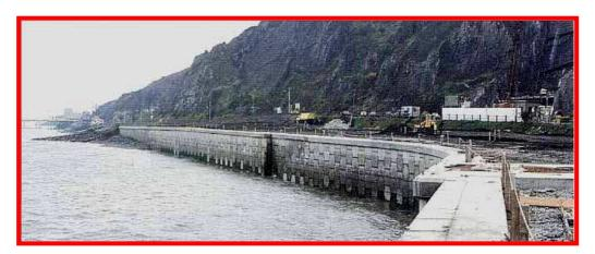
In 1983, a parking area and boat launching ramp were built directly on Reinforced Earth walls at the port of Swansea on the southern coast of Wales in Great Britain.
