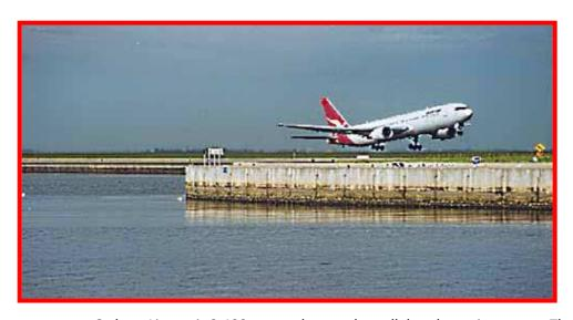
The new runway at Sydney Airport is 2,400 metres long and parallel to the main runway. The vertical seawalls minimise the environmental impact and do not provide a habitat for wading or roosting birds. The total length of walling is approximately 8.5 kilometres, varying in height between 4 and 6 metres and totalling 40,000 square metres. The walls are vertical and in some areas incorporate a wave deflector profile at the top of the wall.
